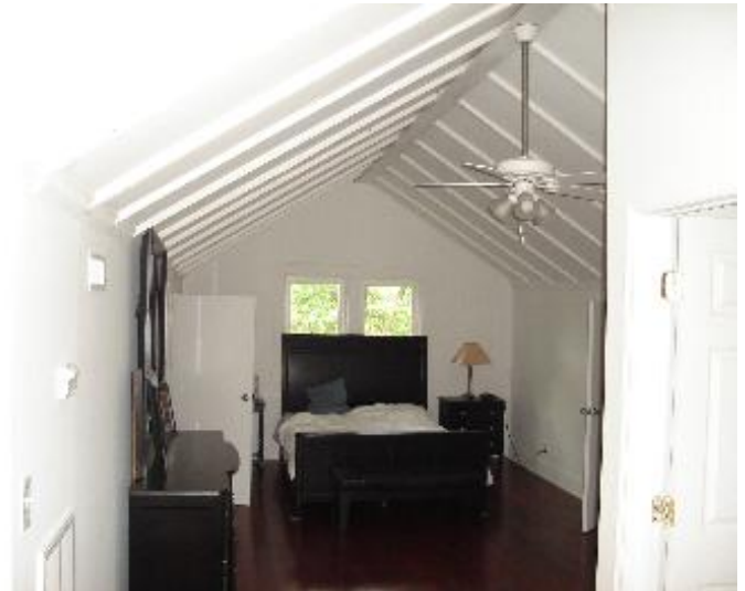
Structural design of the second-floor creates an increase cooling load on HVAC equipment. Construction design must be taken into account when appropriately sizing the equipment. All walls, and ceilings are against unconditioned spaces. There is no attic space above to adequately ventilate the heat above the ceiling.
