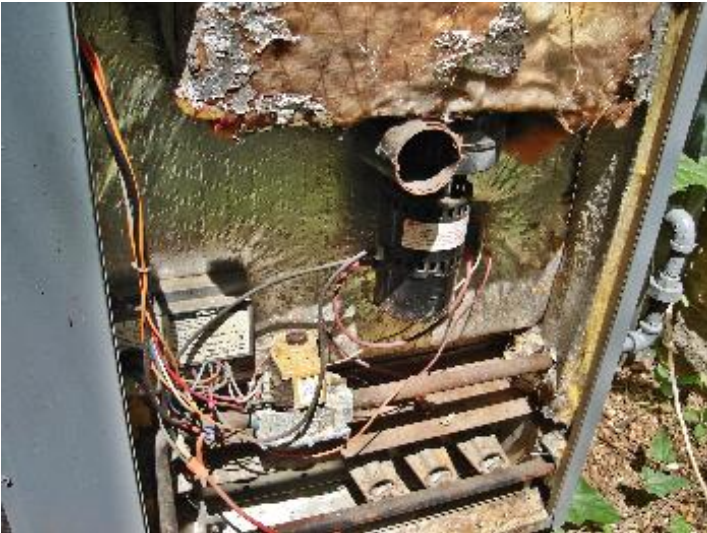
First floor gas compartment condition.
